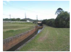
Sydney Water Upper Canal
